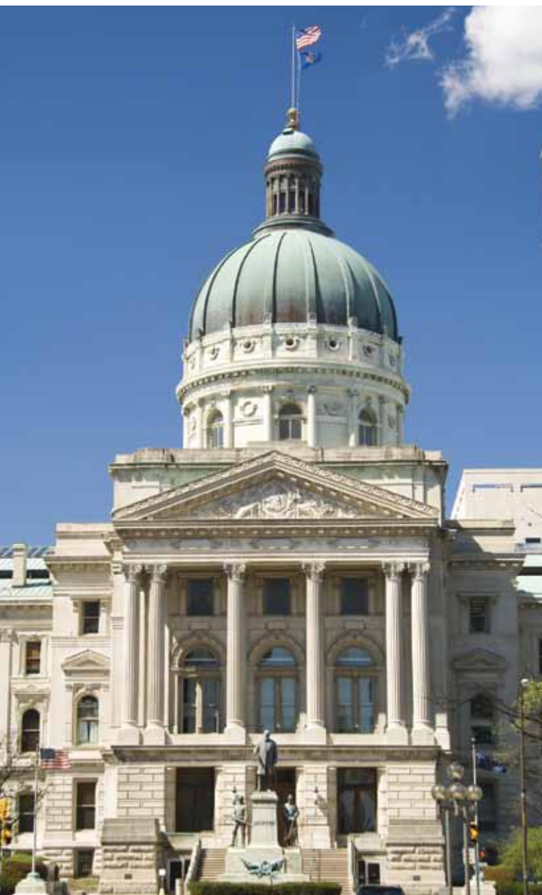
The Indiana State Capitol Building
